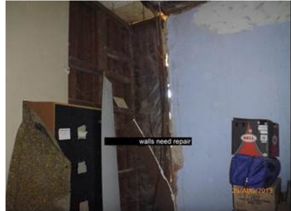
Wall open to outside (2013)
